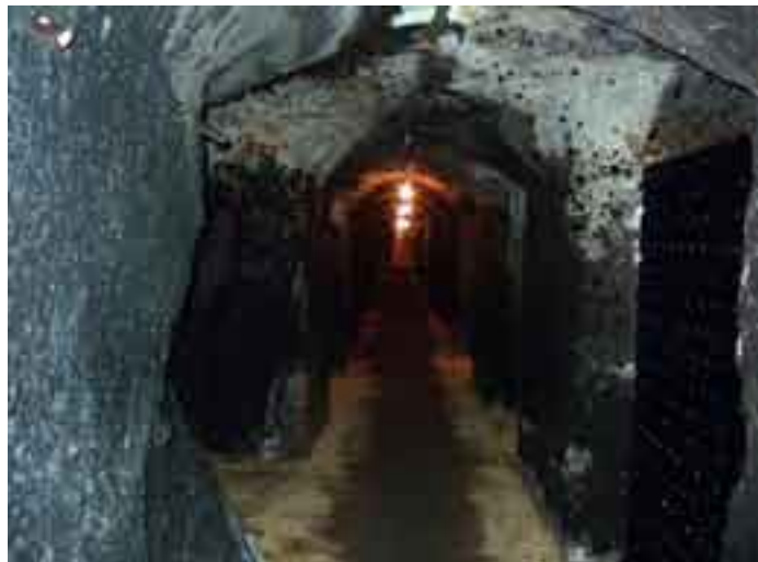
Tunnel showing the decomposed granite walls.
