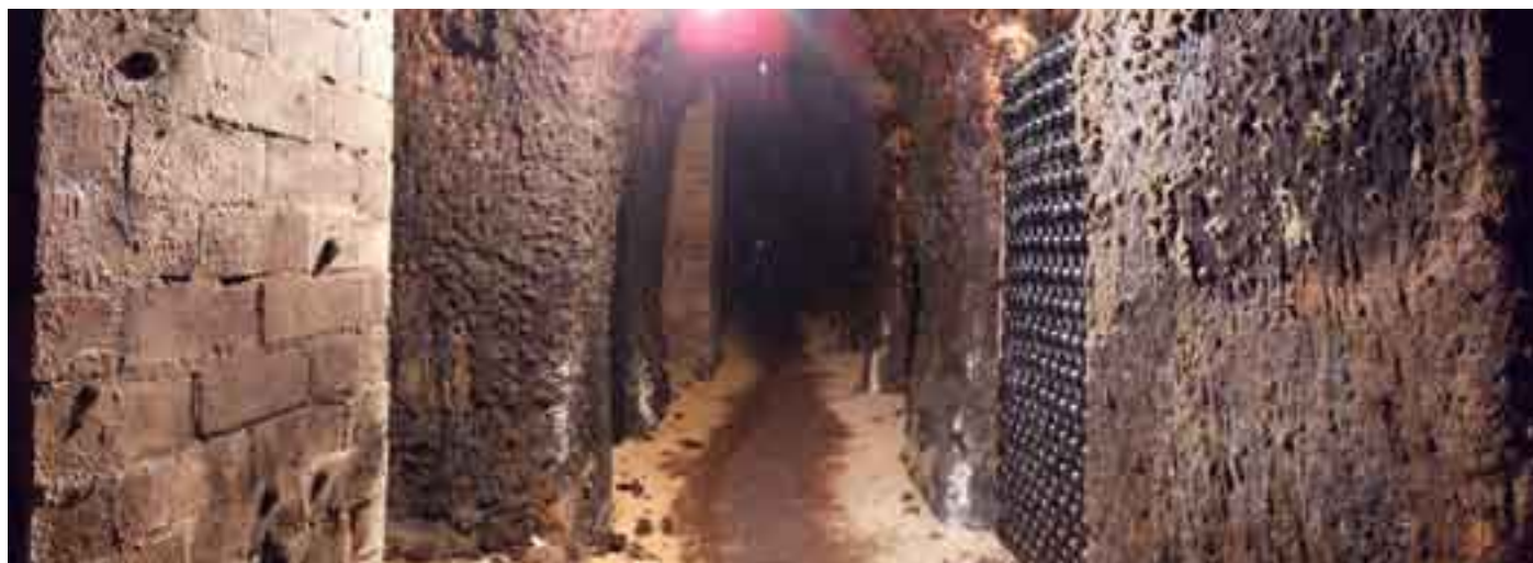
Fungus growing on the walls of Jean Trouette Drive.
